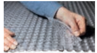
Installing the DURABASE DD 80 ++ double drainage mat with overlap
